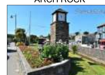
PC3171 PERRANPORTH CLOCK TOWER
